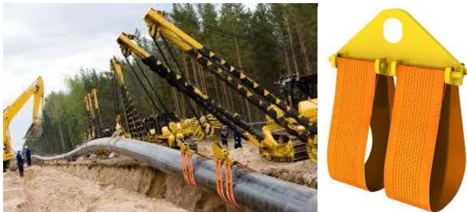
Figure-1. Laying of pipes by means of synthetic textile tapes
