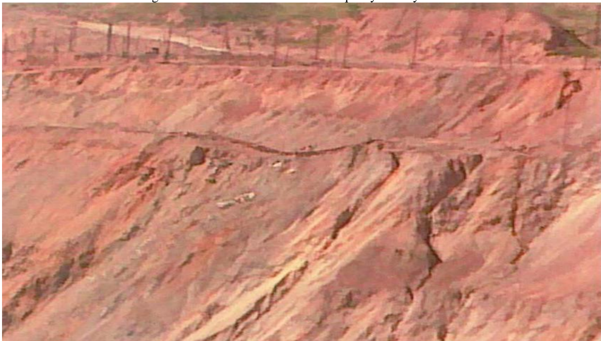
Fig. 2.1. Deformation of the southwestern side of the Kalmakyr quarry.
