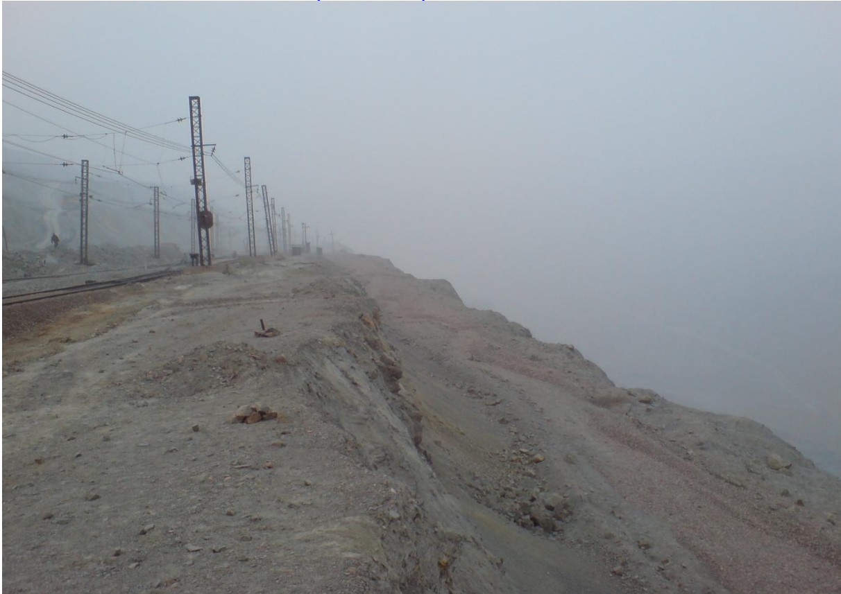
Fig. 2.2. Deformation of the southwestern side of the Kalmakyr quarry.
