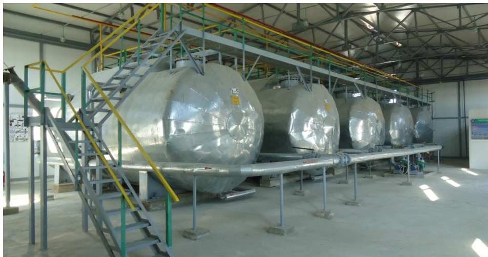
Fig.3. Biogas complex Karaulbazar district of Bukhara region.
