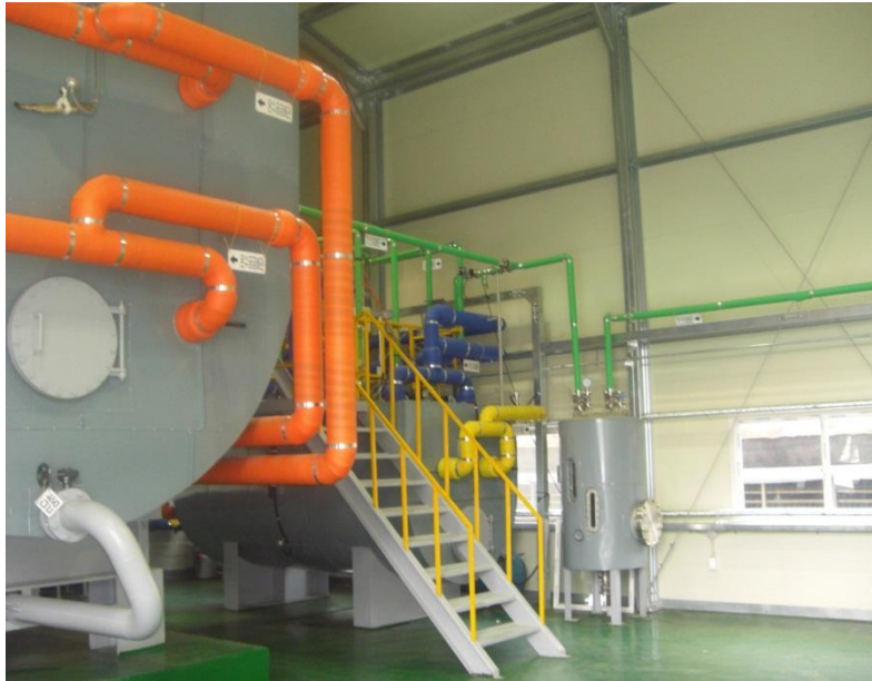
Fig.1. Biogas plant. Seoul
