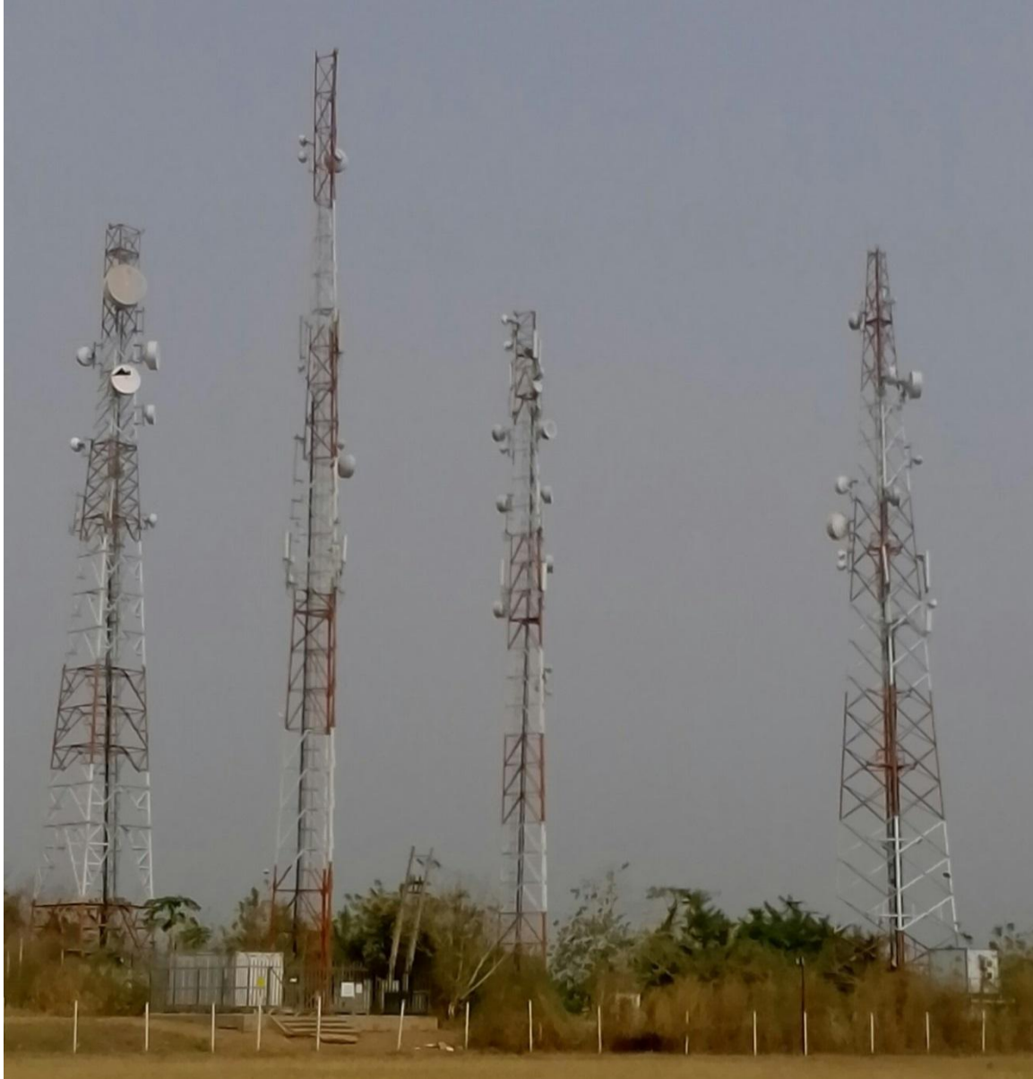
Figure 2.2: Pictorial view of base station at Federal Polytechnic, Ado Ekiti.
