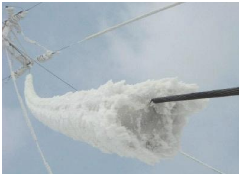
Figure 2. Characteristics of typical wire power lines icing
