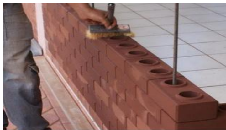
Fig. 1. Laying the "LEGO" brick
