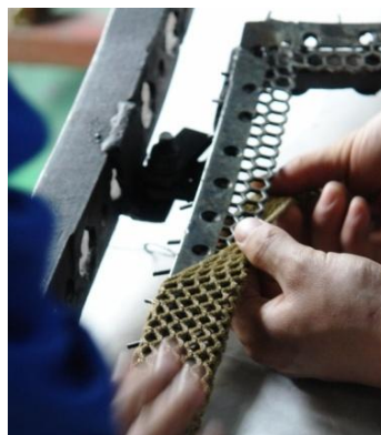
Fig. 7. Fastening the heat-insulating fabric.
