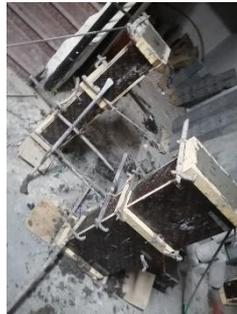
**Fig.4:** Columns casted in wooden formwork.
