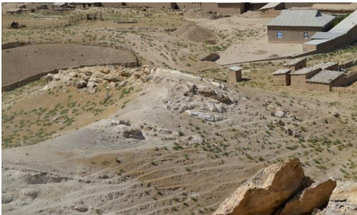
Figure 4. Excavation of clay rocks in Pachkamar section.
