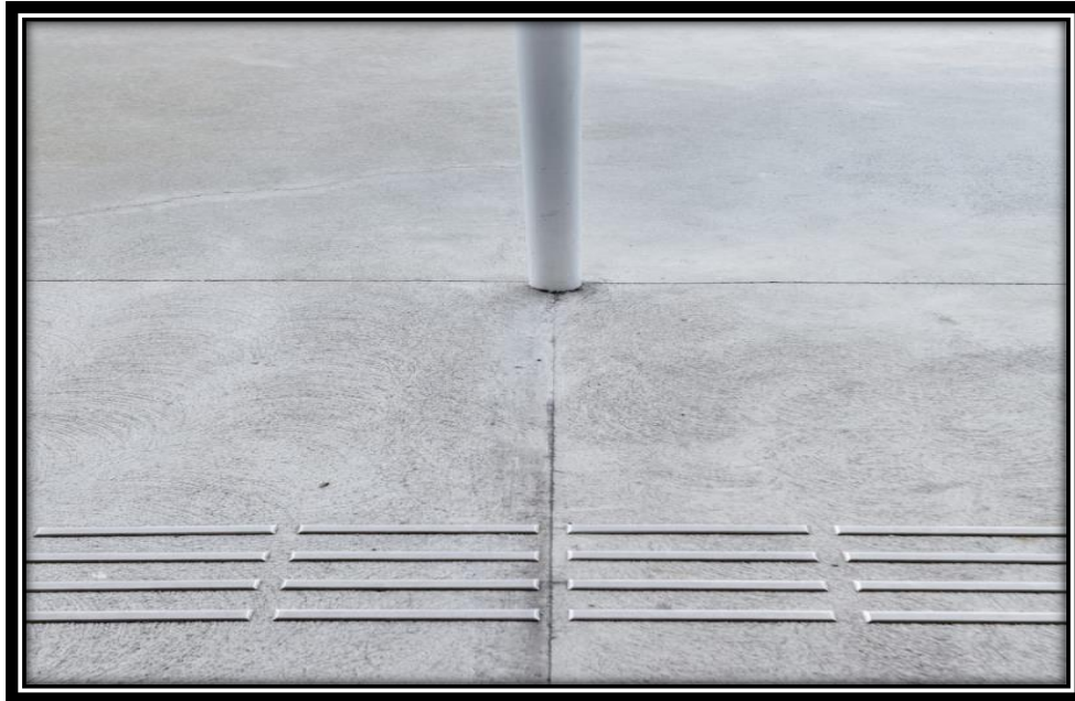
Plate 6: shows the slender and less obvious columns that do not impede passengers from viewing spectacular scenery.
