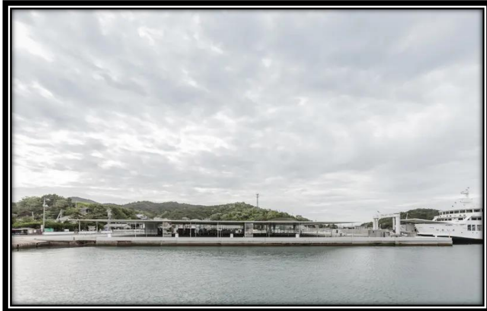
Plate 7: shows the approach view of Naoshima terminal.
