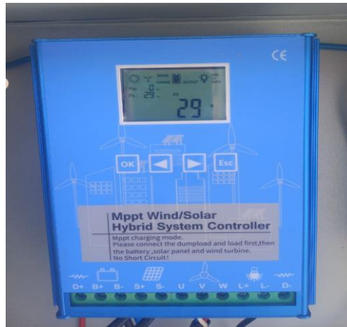
Fig 2. Special Controller for Hybrid System Composed of Wind Turbine and Solar Panel
