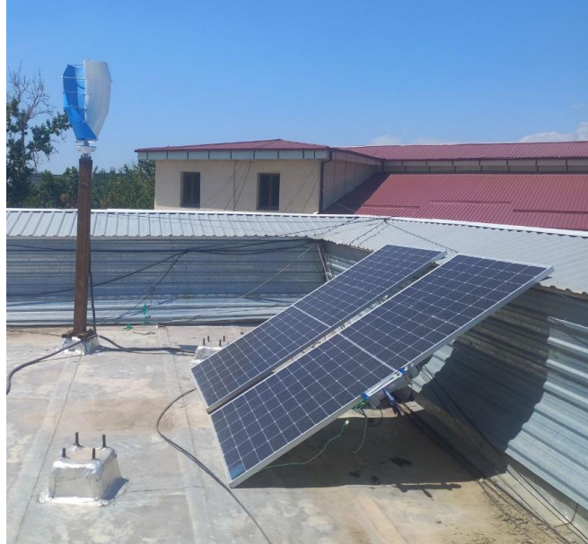
Fig1. Solar-Wind Hybrid System.
