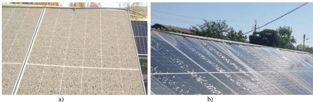
Fig. 3. Surface dusting of solar panels (a) and cleaning technology (b)
