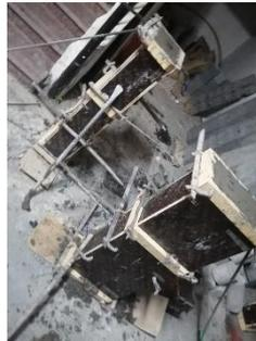
**Fig.4:** Columns casted in wooden formwork.
